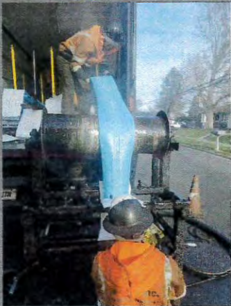
Sewer Lining Installation
