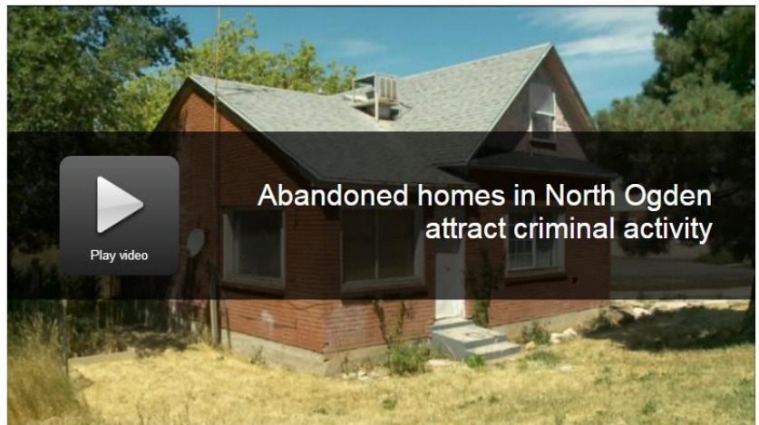
NORTH OGDEN, Utah — They are unsafe, unsightly and condemned.
