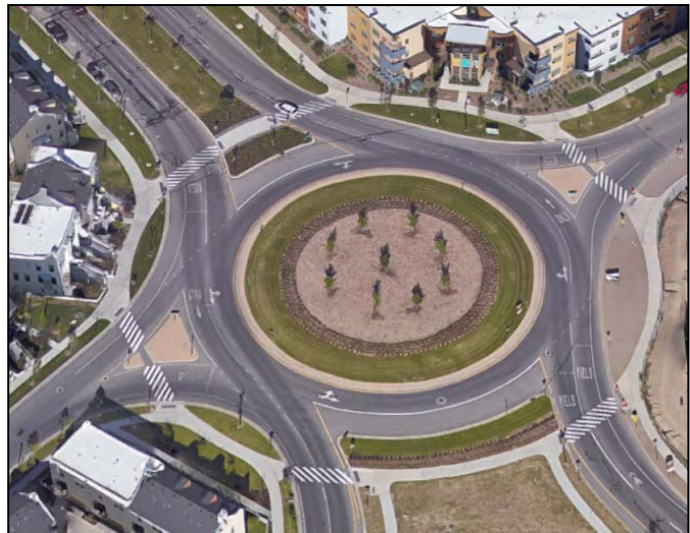
Walkable Roundabout with Skewed Approaches, Daybreak, South Jordan, UT
