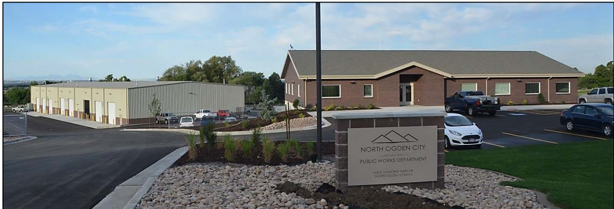
New North Ogden Public Works facility
