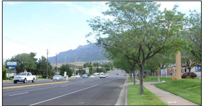
Current View North on Washington Boulevard Approaching 2600 North Intersection
