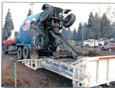
Figure 13. Mixer truck being washed out into a roll-off bin
