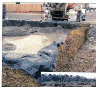
Figure 9. Hay bale and plastic washout pit
