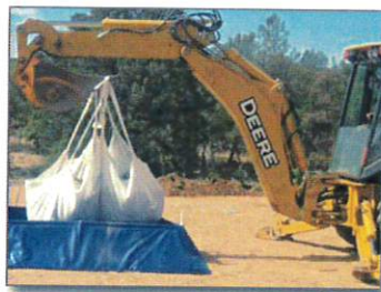
Figure 12. Extracting the concrete solids or gelled washwater
