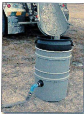
Figure 3. Concrete washout filter
