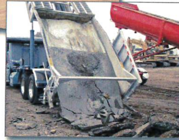
Figure 15. Delivering hardened Concrete to a recycler
